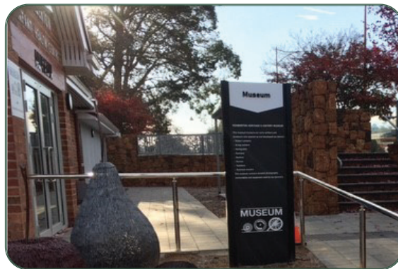
Accessible path and railings at Pemberton Community Hub Balang Miya
