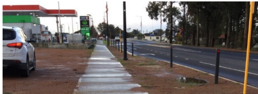
Figure 2-6 South Western Highway
