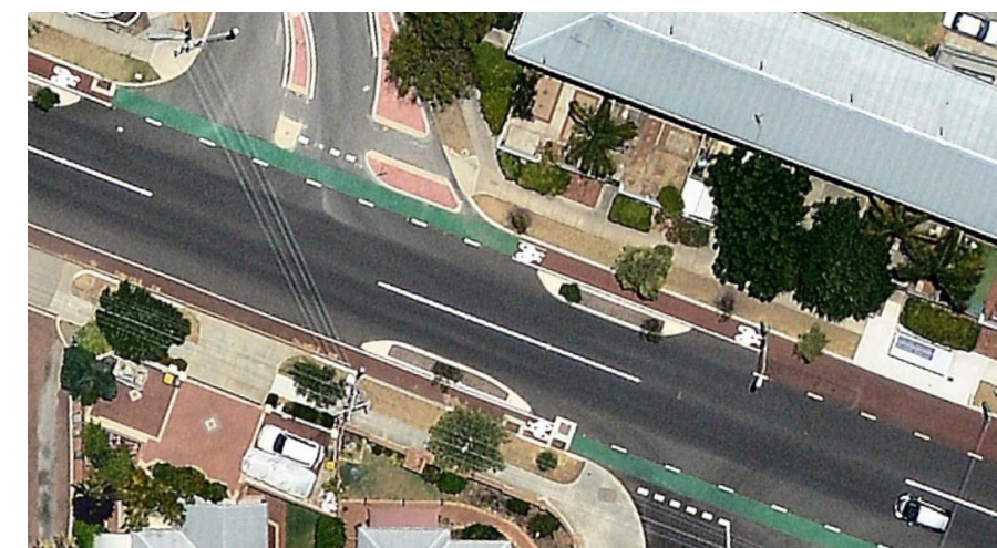
Figure 1-4 Example of dedicated on-street bike lanes Source: Nearmap (2017)
