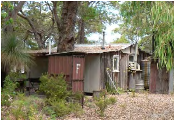
Photo 8: Heavy fuel loading on and surrounding one of the shacks
