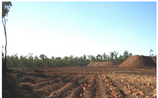
Completed rehabilitation earthworks - Frosty Road (Wolf Tiedemann)→
