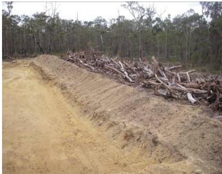
A well laid out topsoil and debris heaps (Jeremy Chick)
