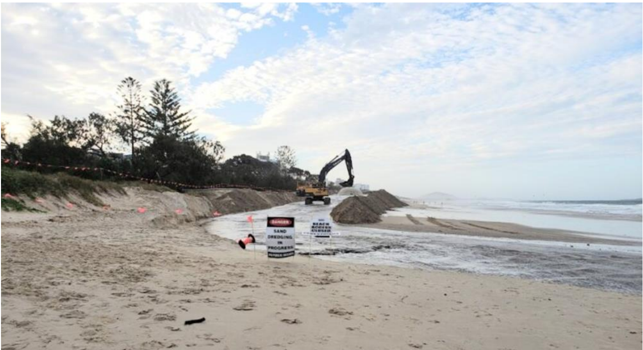
Figure 7-2 Beach nourishment underway at Sunshine Coast, QLD
